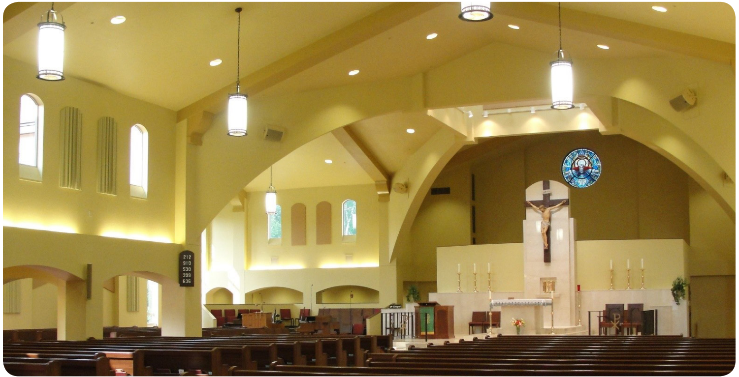
Parallel, reflective side walls and a smooth, flat reflective rear nave wall caused problems. This “after” photo shows the addition of diffusion panels between and below the two windows at the left. Absorption panels are visible on the left front wall. Even larger absorption panels were used on the back wall. Exposed speakers solve the problem of original speakers being housed in wall cavities.
