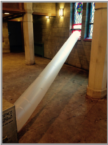
Air vents keep things safe during asbestos abatement.
