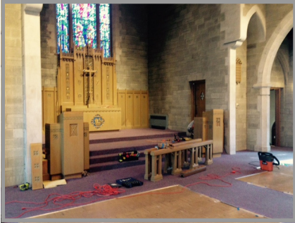
Pews are out; chancel work begins.
