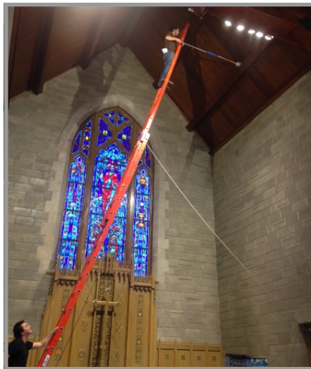
Dusting the ceiling requires courage and a good sense of balance.
