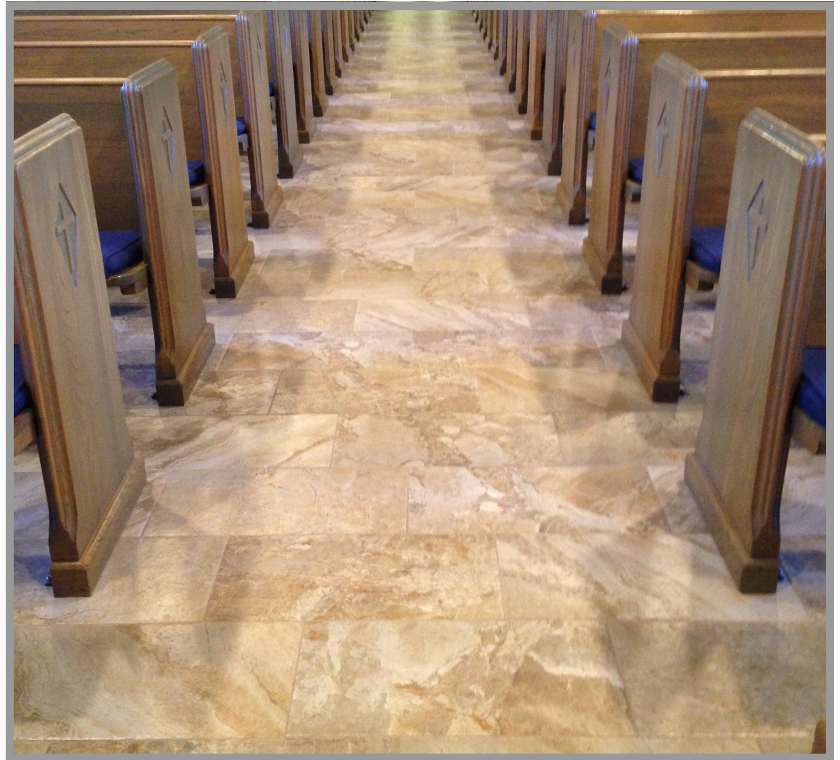
For the hearing disabled, a hearing loop has been installed beneath our new floor.
