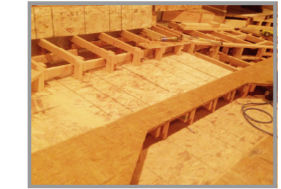
The balcony floor is restructured.
