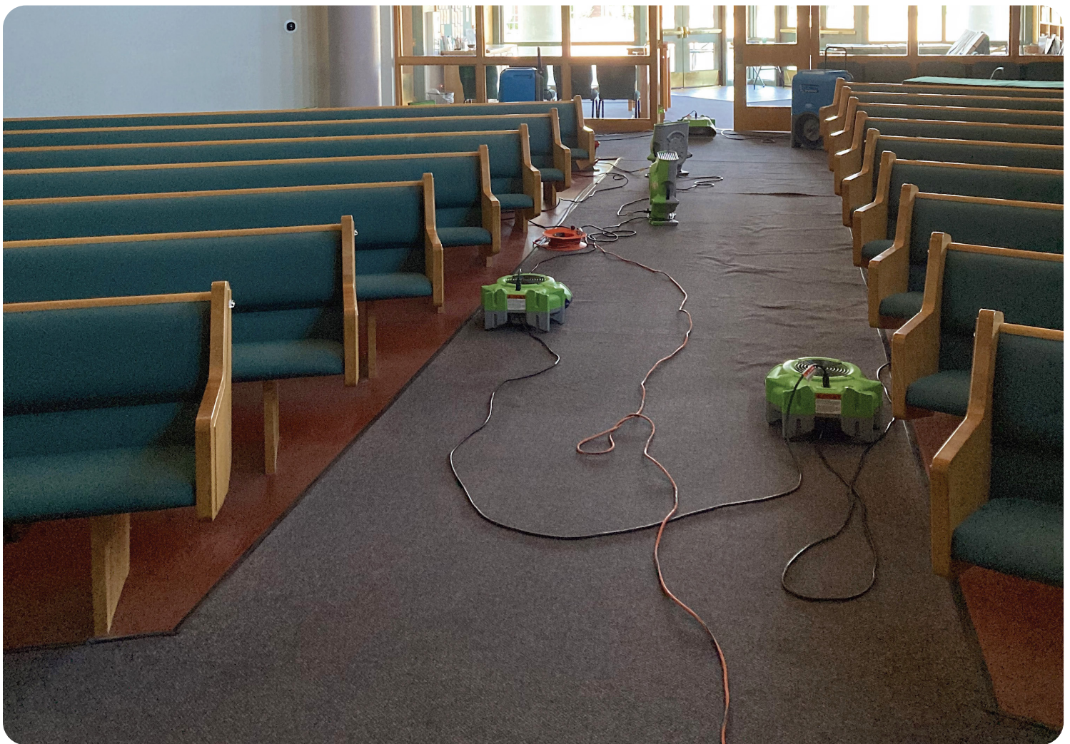
Dark flooring and green pews before the renovation—and after a broken sprinkler flooded the chapel.
