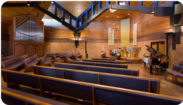
A 2015 renovation removed carpet and polished the concrete beneath, painted the beams, and installed hardwood in the chancel. All photos in this article are from Our Redeemer .
